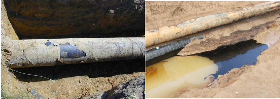
Figure 3-1 Pipelines carrying crude oil
