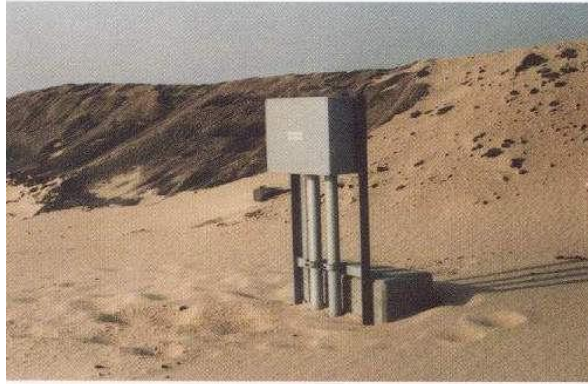
Figure 3-6 The junction box
